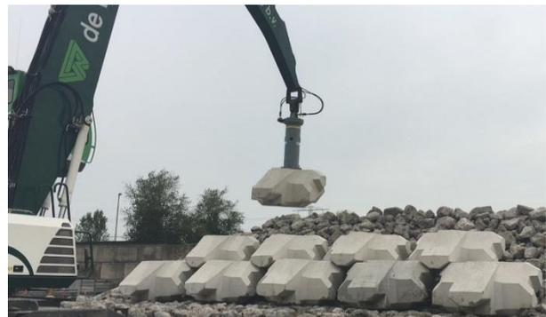
Figure 4: Placement of 6.5ton XblocPlus
