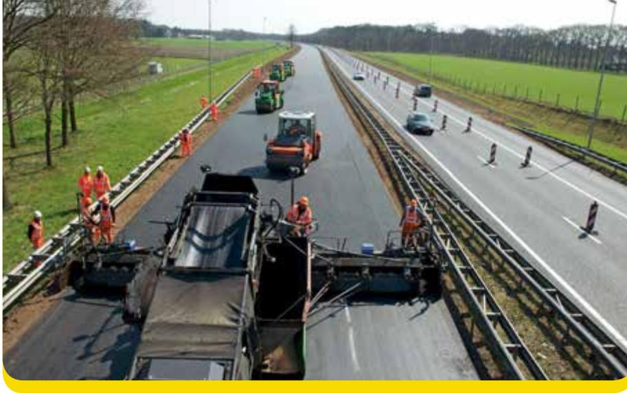
LEFT: The warm asphalt material offers a wider window for compaction
